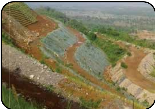
Experiments at the mine to assess the suitability of various dump stabilization methods
