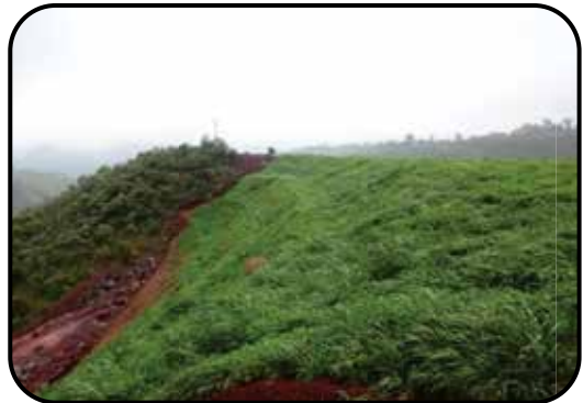
Dump Stabilization at the mine
