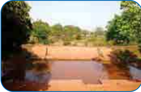
Rain Water Harvesting Structure
