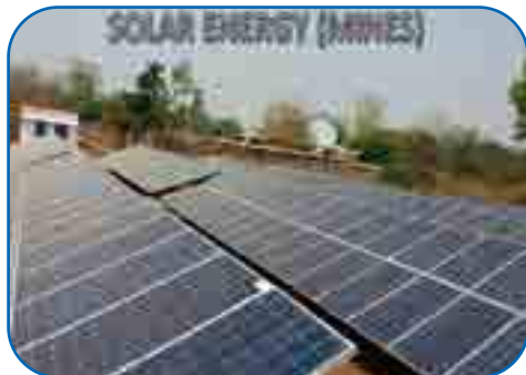
Solar Power Plant installed at mines
