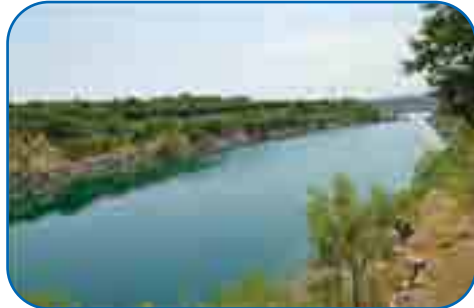
Green Belt development & Water Storage
