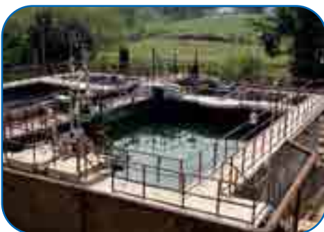
SBR Technology Based STP of 2MLD Capacity
