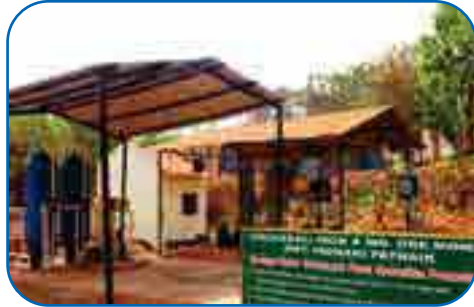
Sewage Treatment Plant
