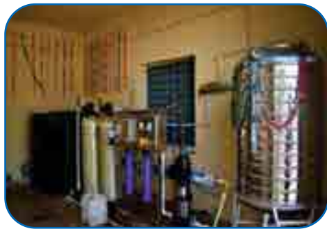
Installed RO Water plant
