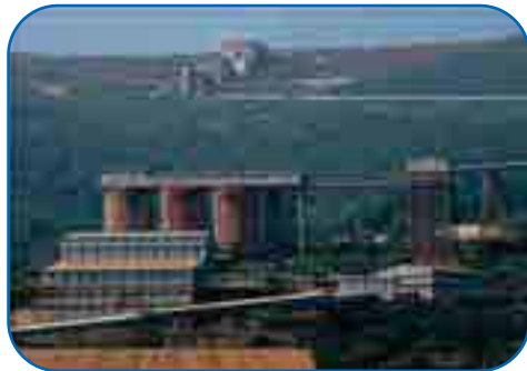
Closed conveyers to prevent dust generation
