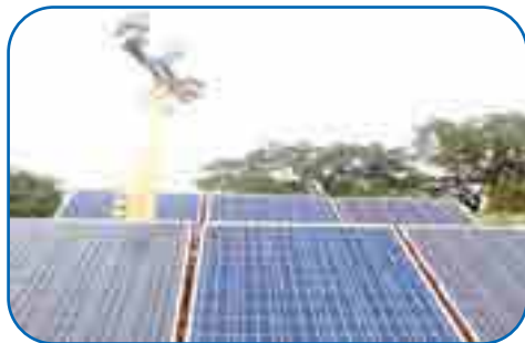
Use of Solar Energy in Mines
