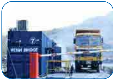
RFID system at entry and exit point
