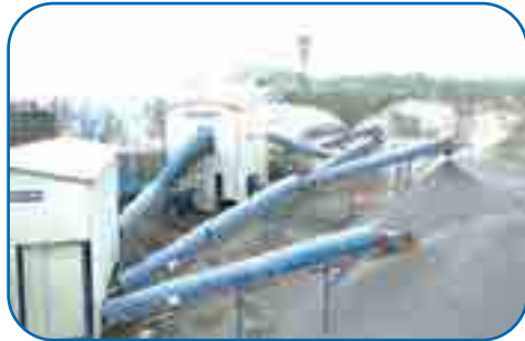
Manufacturing Plant with Dust Extraction System
