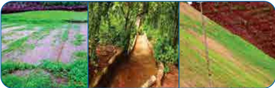
Dump Stabilization with Coir Mat, Vertiver and Grass Seed Applications with proper drainage System
