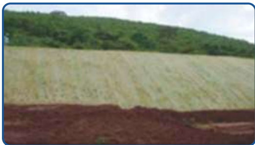
Geo-Coir covering on Dumps
