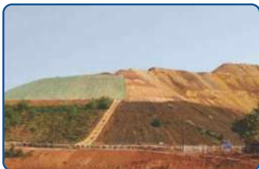
Systematic dump management with coir mat and vetiver
