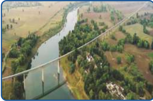
21 km OLBC connecting Mines to Plant
